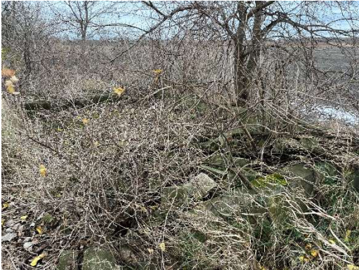
View of Building Foundations Near Dilapidated Silos
