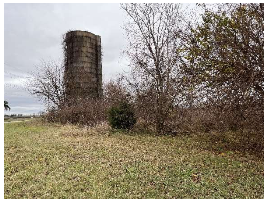
View of Dilapidated Silos Facing South on 02-19-200-006
