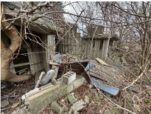
View of Building Remnants Near Dilapidated Silos
