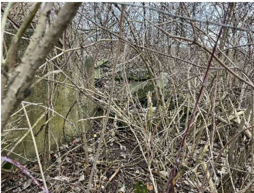
View of Building Foundations Near Dilapidated Silos
